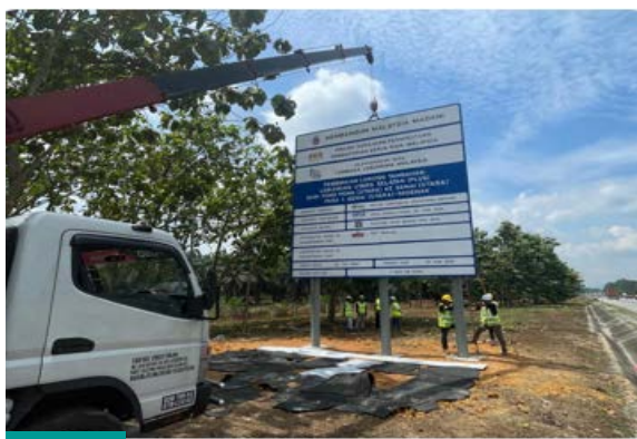
Kerja Pemasangan Papan Tanda Projek di KM 45.2 Arah Selatan Installation of Project Signboard Installation Work at KM 45.2, Southbound
