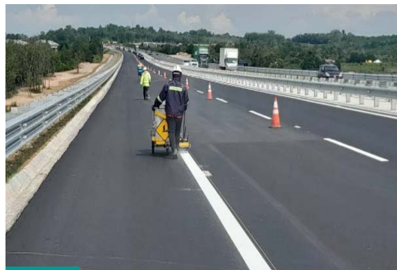
Penandaan garisan jalan di KM 123.6 arah timur barat Road line marking at KM 123.6 east-west
