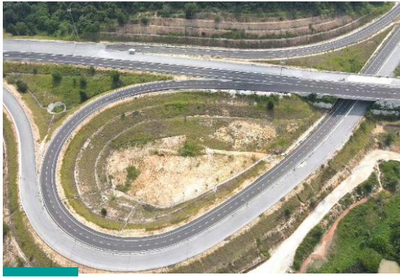
Persimpangan Hulu Langat Hulu Langat Interchange
