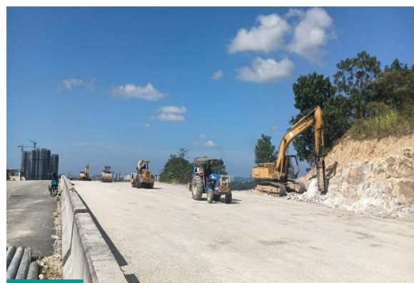
Ramp 1B Ch 330 LHS : Kerja-kerja pemecahan batu dijalankan bagi kerja longkang. Ramp 1B Ch 330 LHS : Rock breaking works are being carried out for the drainage works.
