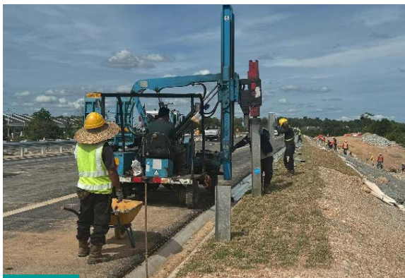
Pemasangan penghadang jalan di KM 123.7 arah barat Installation of roadblocks at KM 123.7 westbound
