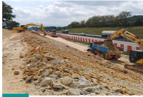
Kerja Pemotongan Cerun di KM 42.9 Arah Selatan Slope Cutting Works at KM 42.9, Southbound
