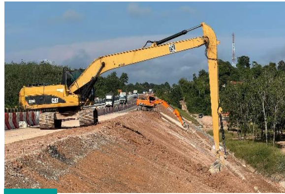
Kerja pelarasan cerun di KM 123.6 arah timur barat Slope adjustment work at KM 123.6 east-west
