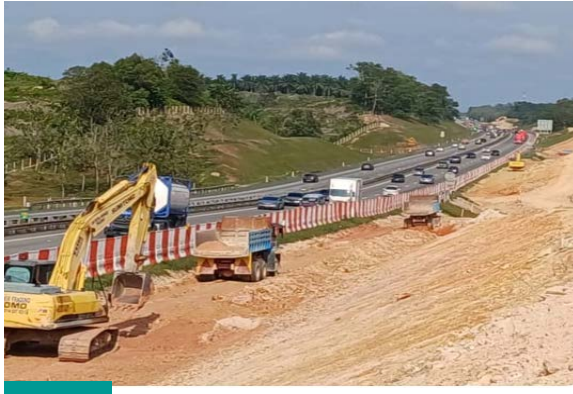
Kerja Pemotongan Cerun di KM 43.4 Arah Selatan Slope Cutting Works at KM 43.4, Southbound
