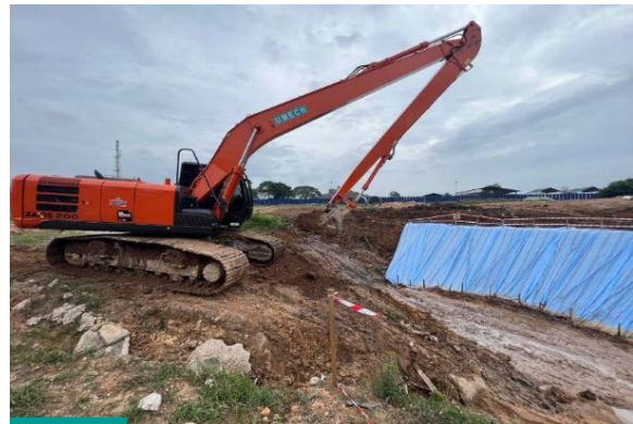
Kerja Remove & Replace Tanah di Kawasan Culvert KM 41.8 Arah Selatan Soil Removal & Replacement Works at Culvert Area, KM 41.8, Southbound
