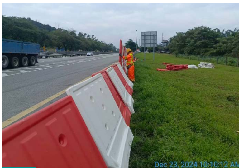
Kerja Pemasangan Peralatan Traffic Management Plan (TMP) di KM 33 Arah Selatan Installation of Traffic Management Plan (TMP) Equipment at KM 33, Southbound
