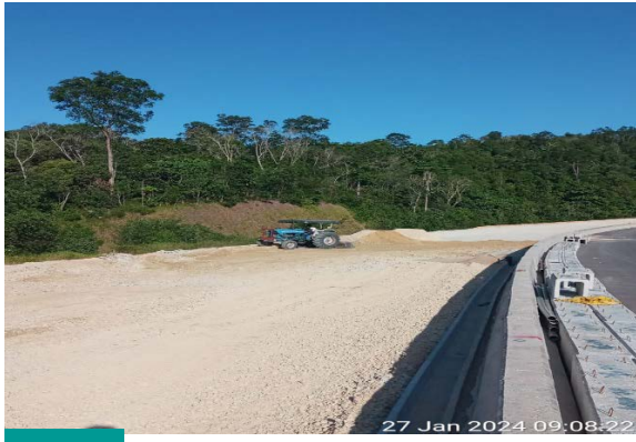
Ch 12530 ke Ch12390/ LHS: Kerja-kerja penambakan sedang dijalankan Ch 12530 to Ch12390/ LHS: Reclamation works are underway
