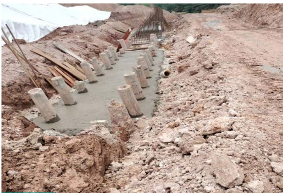
Asas tapak konkrit di KM 117.7 arah barat Concrete foundation at KM 117.7 westbound
