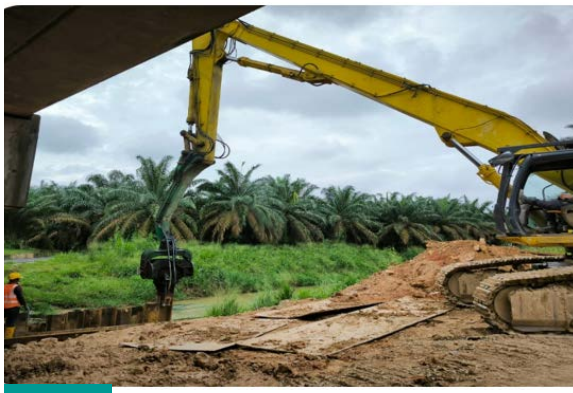
Kerja Pemasangan Temporary Sheet Pile di Kawasan Bridge 3 (KM 35.1) Temporary Sheet Pile Installation Works at Bridge 3 Area (KM 35.1)
