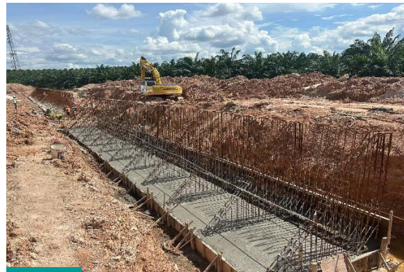
Asas tapak konkrit untuk tembok penahan cerun di KM 117.8 arah barat Concrete foundation for slope retaining wall at KM 117.8 westbound
