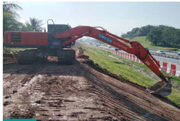
Kerja Site Clearing di KM 35.6 Arah Selatan Site Clearing works at KM 35.6, Southbound
