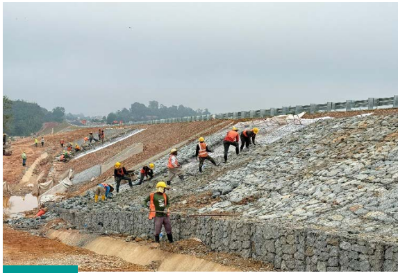
Pemasangan 'gabion mattress' di KM 123.5 Installation of 'gabion mattress' at KM 123.5
