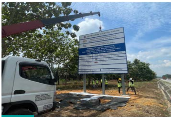
Kerja Pemasangan Papan Tanda Projek di KM 45.2 Arah Selatan Installation of Project Signboard Installation Work at KM 45.2, Southbound
