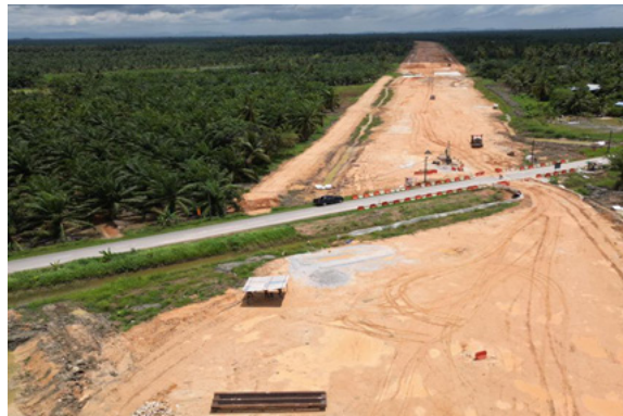
Pembinaan jejambat di Seksyen 7 (Jalan Tanah Serong). Construction of a flyover in Section 7 (Jalan Tanah Serong).
