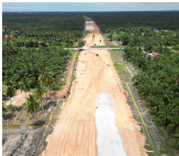
Kerja-kerja tanah di jajaran utama lebuhraya di Seksyen 7. Land works on the main alignment of the highway in Section 7.
