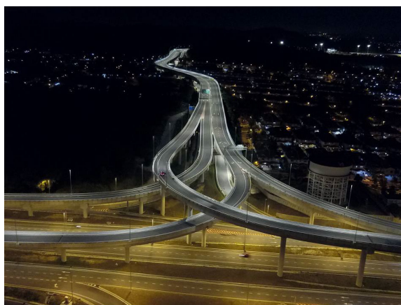
Persimpangan Puncak Perdana di Persiaran Mokhtar Dahari Puncak Perdana Intersection at Mokhtar Dahari Drive
