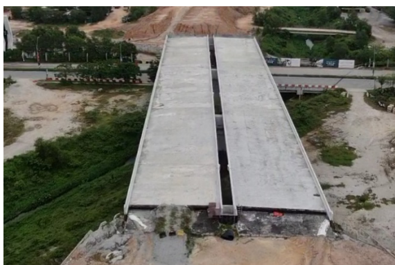
Pembinaan jambatan berhampiran Projek Cybersouth. Bridge construction near the Cybersouth Project.
