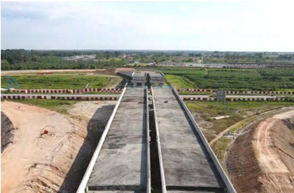
Pembinaan persimpangan Banting (Seksyen 1). Banting Intersection construction (Section 1).
